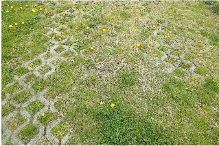
Figure 25: Grass pavers allow water to seep away and enable low vegetation – they have many advantages over sealed surfaces.
